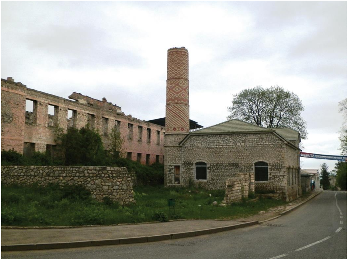
Images 5–7: Saatli Mosque, Shusha ( XVIII century. The interior of the mosque was completely demolished and its minaret was partially destroyed after the occupation of Shusha in 1992 )
